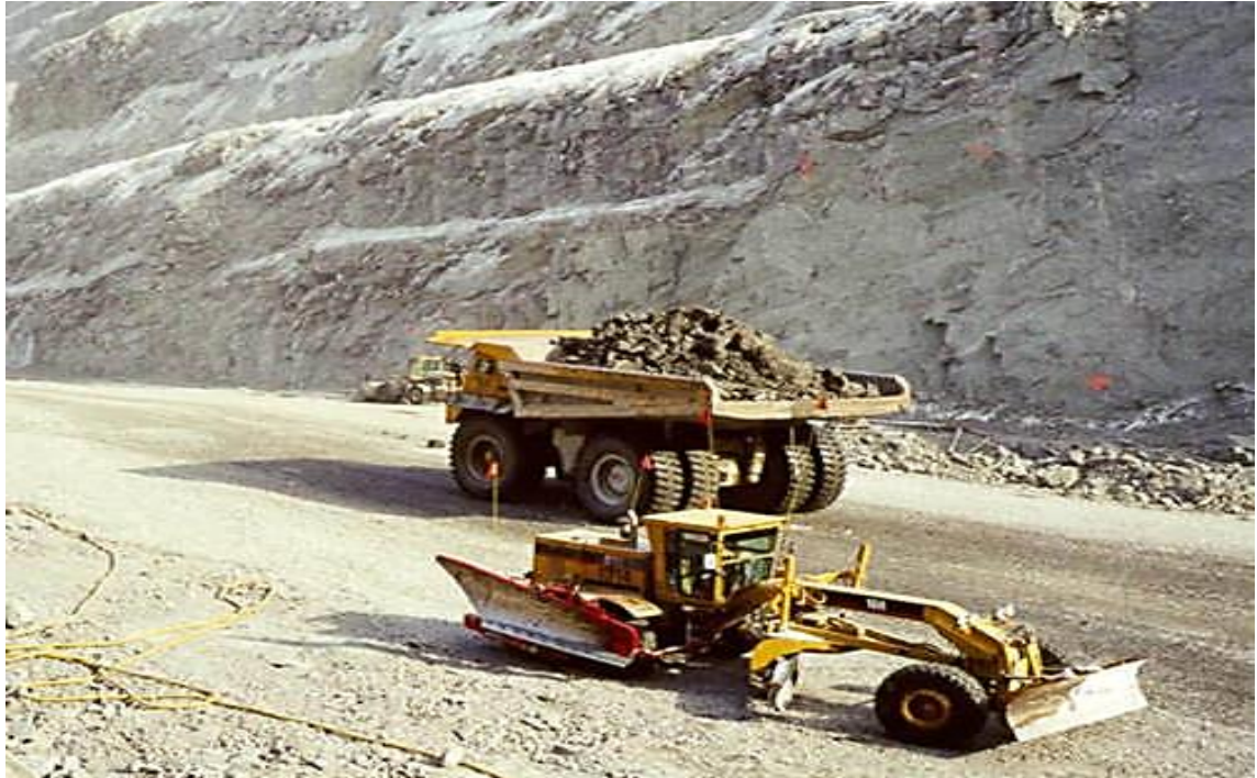
Maintenance of Haul Road in Progress
