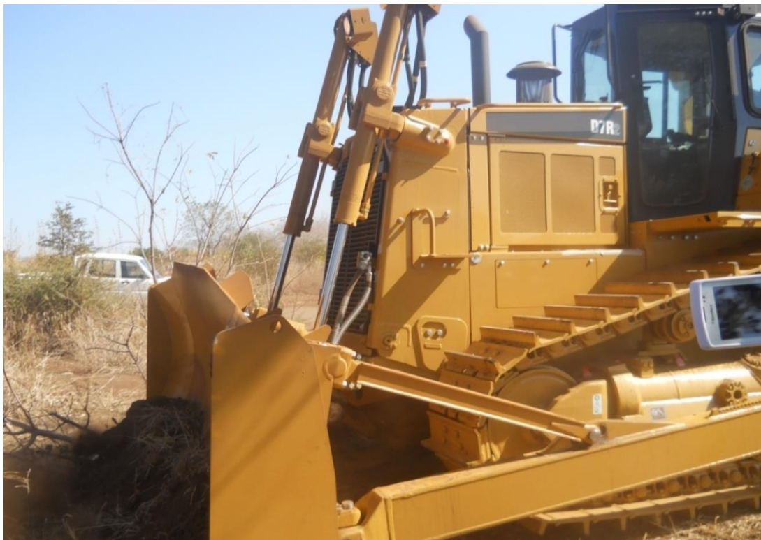
D7R in Grubbing Operation
